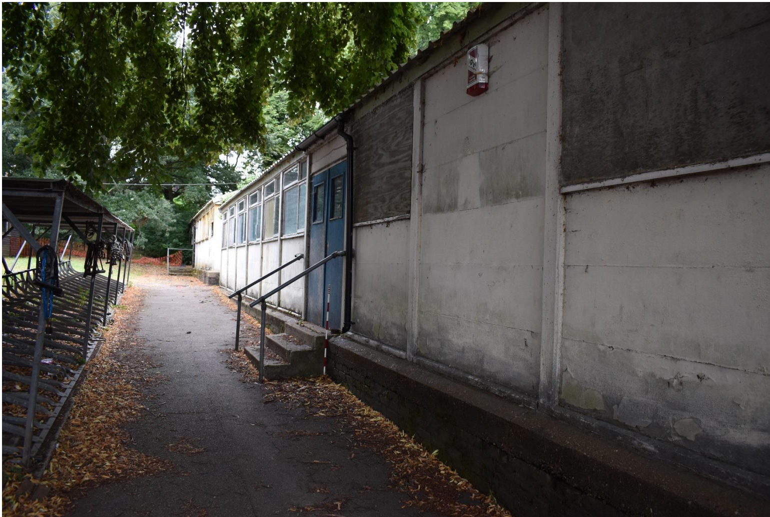
Plate 10: View along the front of the 1940s classrooms (facing SW).
