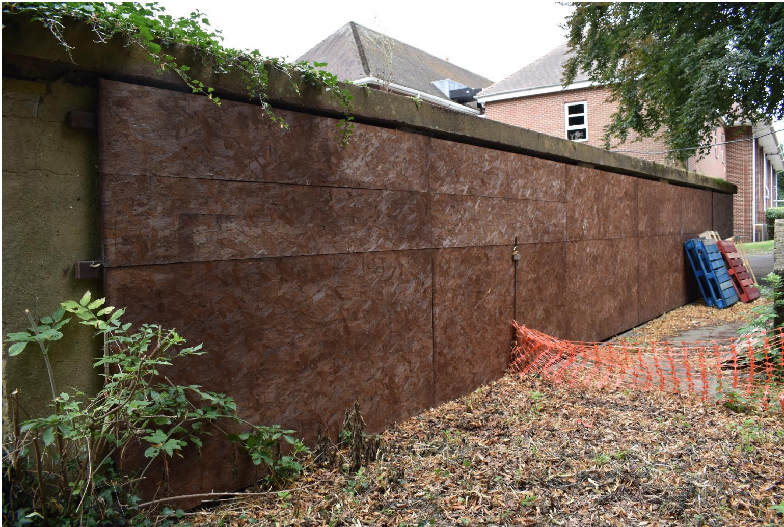
Plate 11: View of the air raid shelter (facing E).
