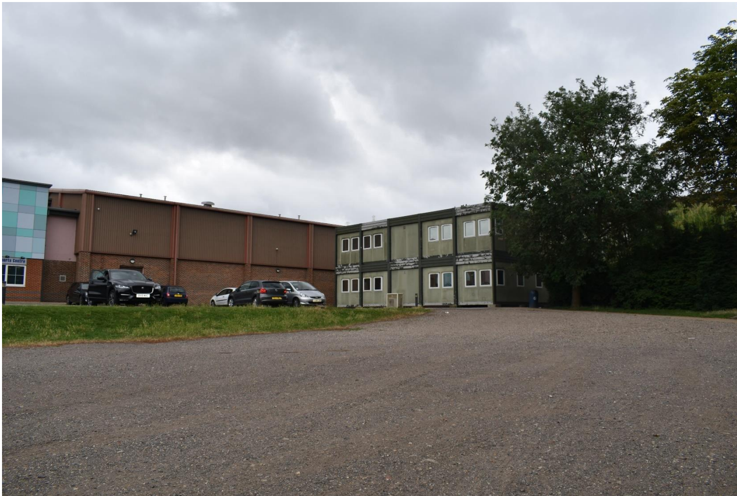
Plate 18: View across the site of the new English block proposed development (facing S).
