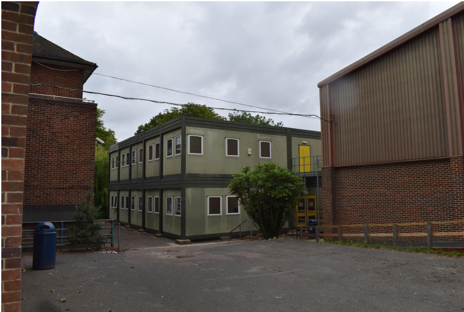
Plate 17: View towards the existing 8 block mobile classrooms (facing NW).
