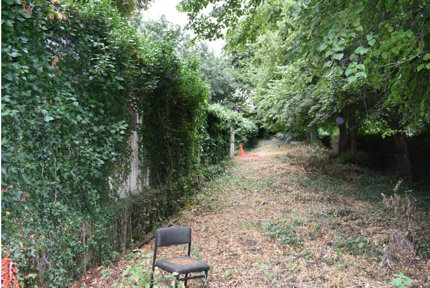
Plate 9: View along the rear 1940s classrooms (facing SW).
