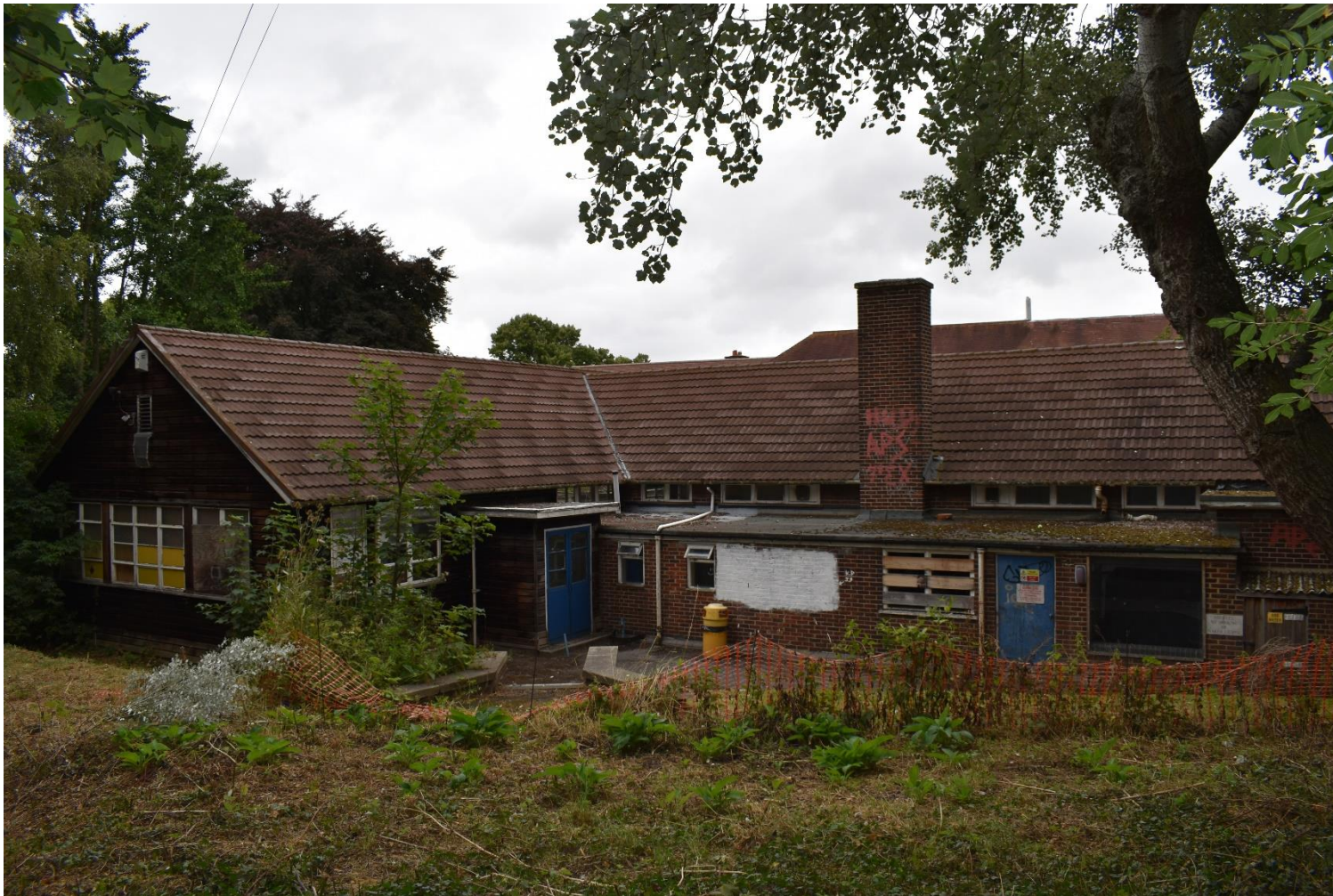
Plate 13: View of the existing canteen (facing N).
