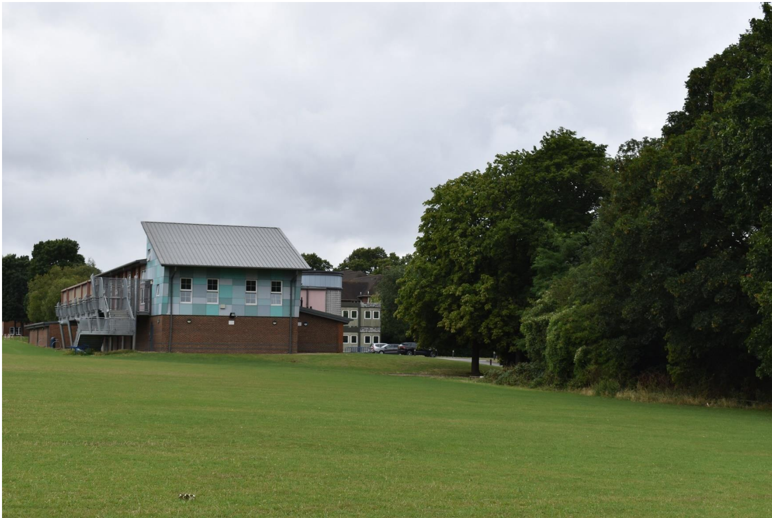
Plate 22: View across the area where the car park is proposed to be extended (facing SW).
